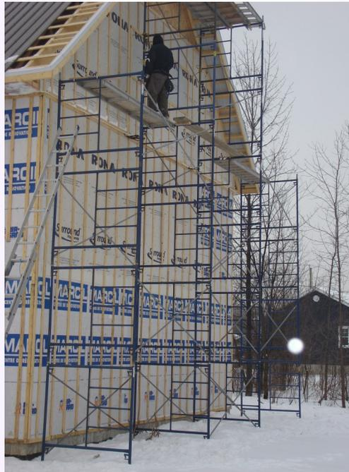
*This scaffold has inadequate planking, missing braces no guardrails and should be tied into the structure*
